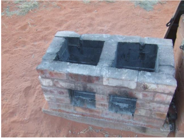
Figure 5. Resistant fire-brick stove (Photo Absalom Vilho)
